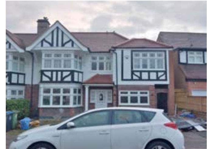
Figure 14: House on Briar Road
