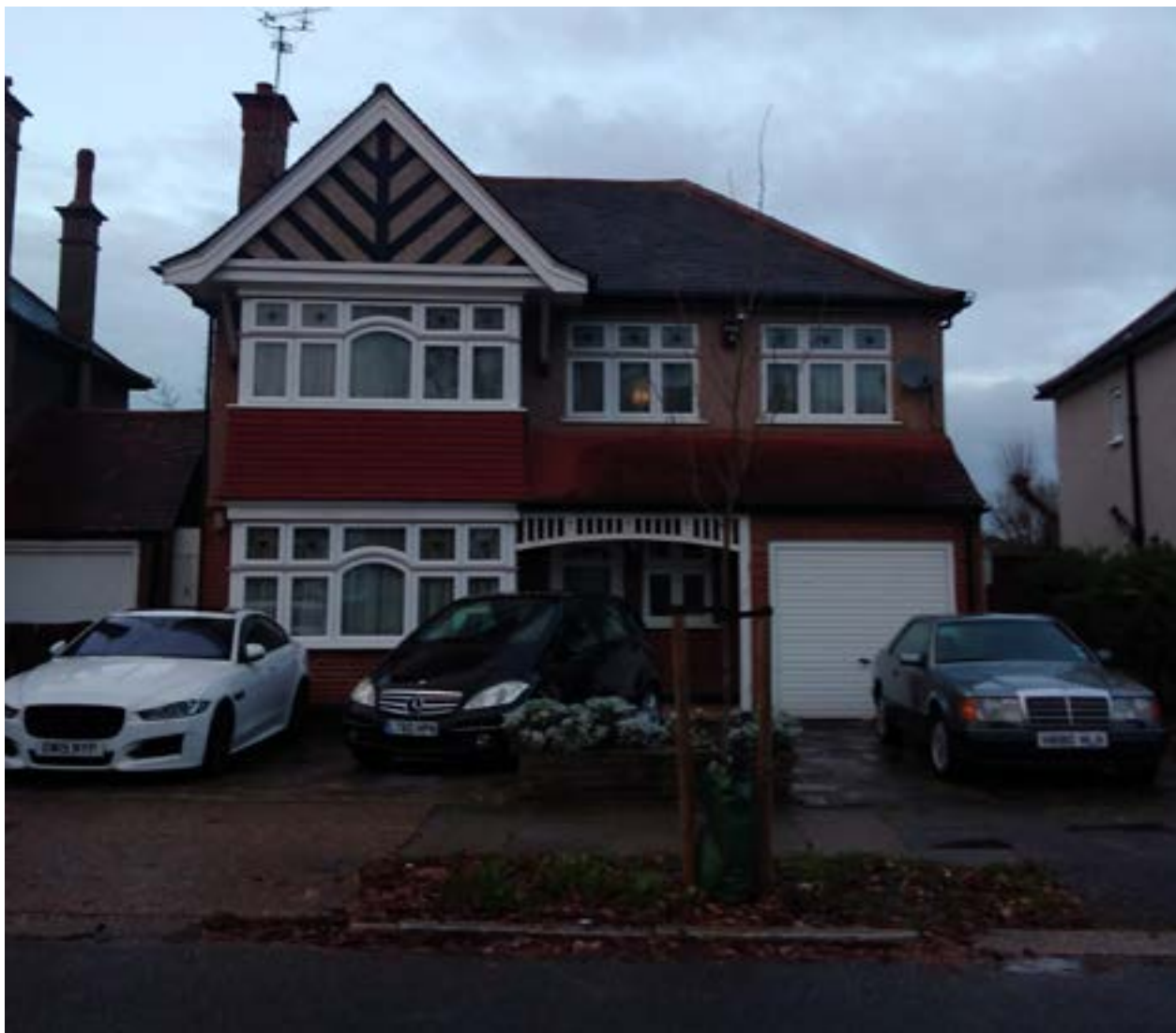
Figure 16: House on Briar Road
